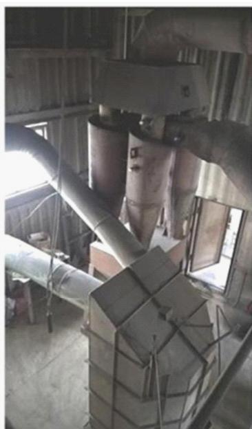
**Fig. 1:** Group cyclone TsN-15-500-4, Wholesale generating company OGK-2, SDPP; top view: cyclone (above), silos (below)
